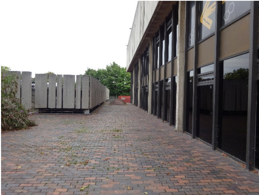
Pic 18: Empty, but paved, space adjacent to Beecroft Art Gallery, Victoria Avenue
