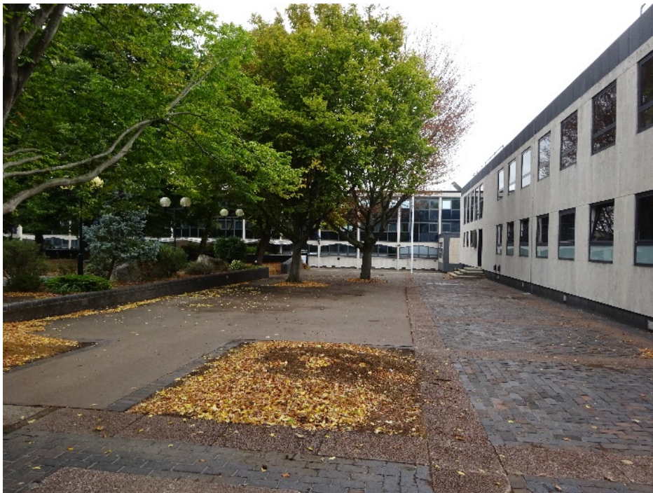
Pic 19: Empty planting space, Courthouse, Victoria Avenue
