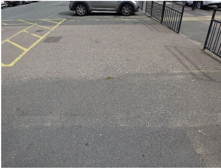
Pic 13: Unused space, York Road car park
